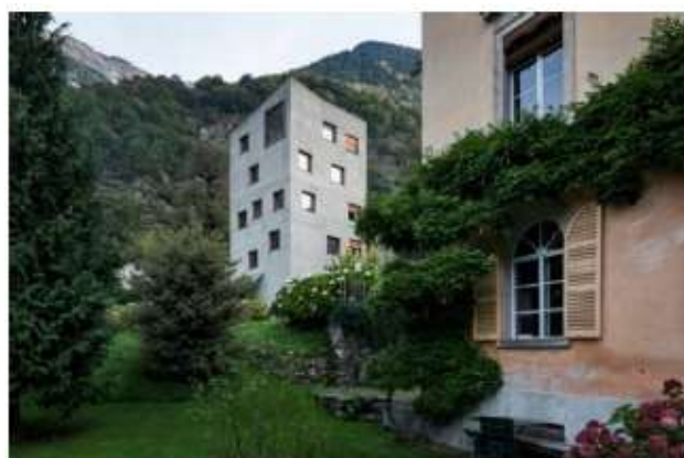
Illustr. 5: Villa Garbald, Castasegna, nouvelle construction arch. Miller e Maranta, 2004 (© Christian Beutler/Keystone)
